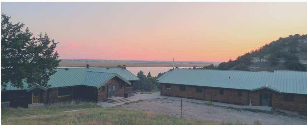
After many years, Goodall Lodge and Gainesforth Resource Center (and other buildings) got new metal roofs in 2020. Photo by John DeLong
